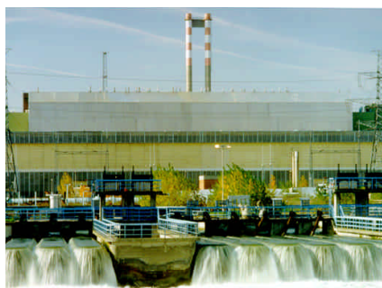
The nuclear power plant in Paks, Hungary.
